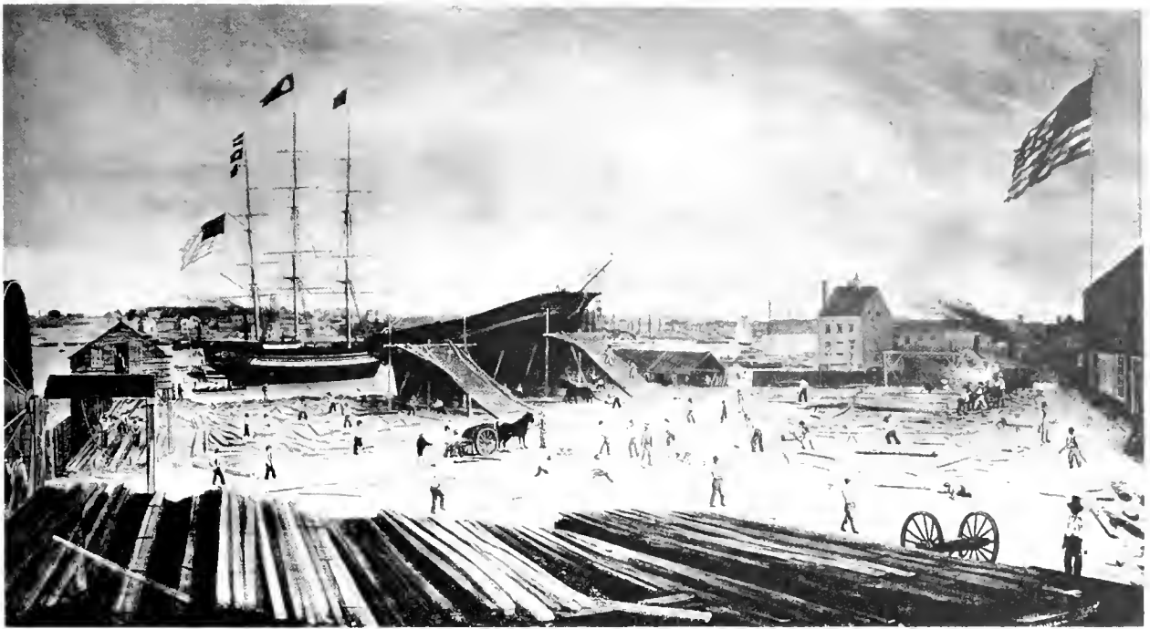
SMITH & DIMON SHIPYARD, NEW YORK, ABOUT 1831, FROM A CONTEMPORARY PAINTING. This firm was then a leading builder of packet ships, and later built Rainbow , Sea Witch and other famous clipper ships. A treadmill can be seen at the extreme left and a steam box at the extreme right. (Smithsonian photo 32914-C.)
